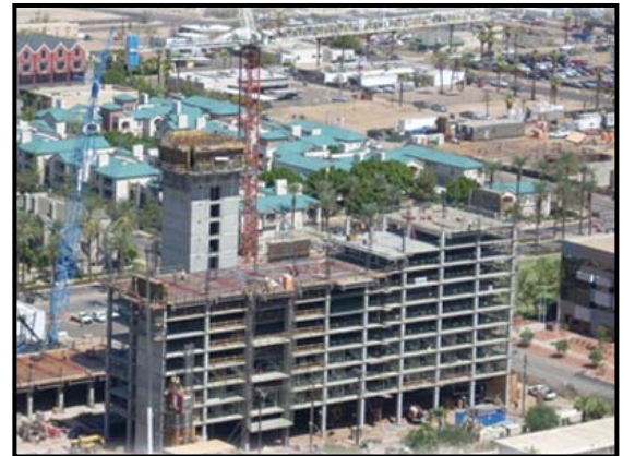
Arizona State University - Taylor Place Student Housing Austin Commercial / Suntec Concrete, 2007 One Peiner SK415 Tower Crane, 75 m jib, 61 m height
